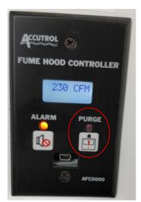
**Verify Proper Hood Airflow.** All hoods should have an airflow indicator that informs the user if the hood is working properly. The indicator readsout in feet per minute, and will alarm when the airflow is not satisfactory. If the airflow monitor is not working, promptly report this or any hood that is not functioning properly (e.g., continuous low flow < 80 fpm while working). The sash should be closed and the hood "tagged" and taken out of service until repairs can be completed.
